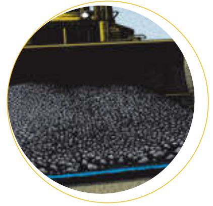
Propex heavy weight nonwoven geotextiles allow the construction of landfill drainage layers without fear of liner damage.
