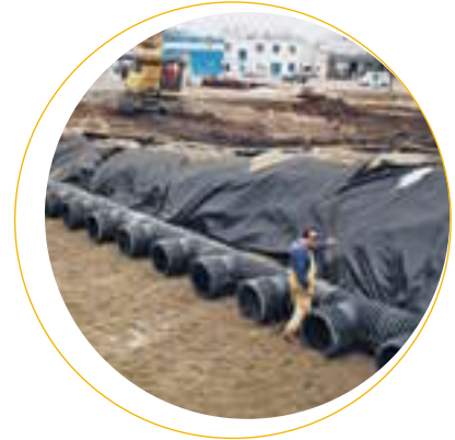
Underground retention/detention systems use Hancor large diameter pipe and Propex geotextiles to effectively control storm water runoff.
