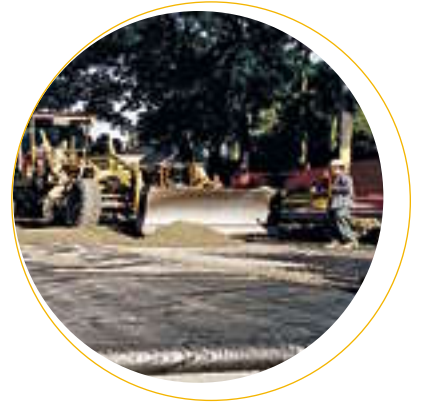
Propex "ST" series of woven geotextiles can reduce aggregate thickness in unpaved roads by as much as 50%.
