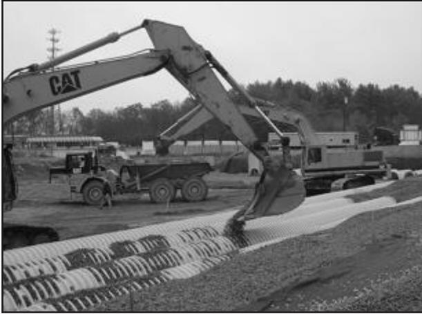
Carefully ladle 3/4-2" (20-50 mm) clean, crushed, angular stone over the centerline of the chamber row.
