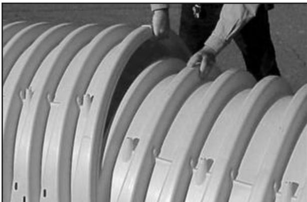
Construct the chamber bed by overlapping the chamber's end corrugations.
