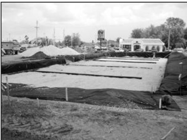
Filter fabric and underdrains installed.
