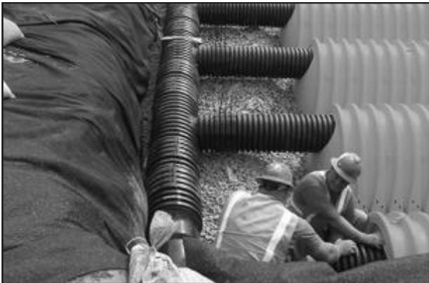
24" - 18" (610-457 mm) reducers installed to stay within the 25" (635 mm) maximum OD limit for the SC-740.
