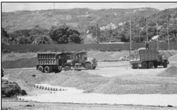
A minimum of three feet (914 mm) cover is required for trucks to dump stone. (See page 7, Section 4)
